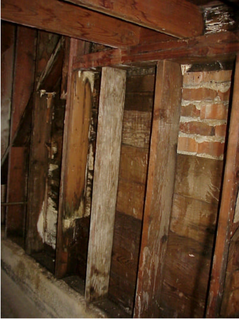
Under Front Stairs
